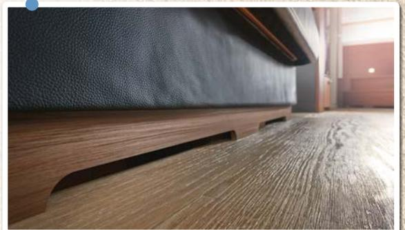
Convector heaters in the double floor protect all the fittings from cold weather. The double floor also serves as a storage heater and gives off heat to the floor similar to underfloor heating. Fully functional underfloor heating is available as an additional optional extra.
