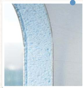
We use aluminium on the outside and styrofoam on the inside, based on the sandwich principle, so that the walls don't conduct either heat or cold.
